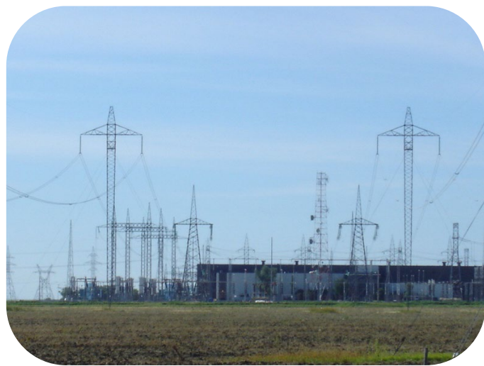
Figure 6 - Long distance High Voltage Direct Current (HVDC) lines carrying hydroelectricity from Canada's Nelson River to a converter station where it is converted to AC for use in southern Manitoba's grid. [Wikimedia. Photo by J. Lindsay, CC BY-SA 3.0]
